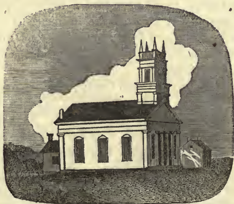
St. Stephen's Church, North Castle
